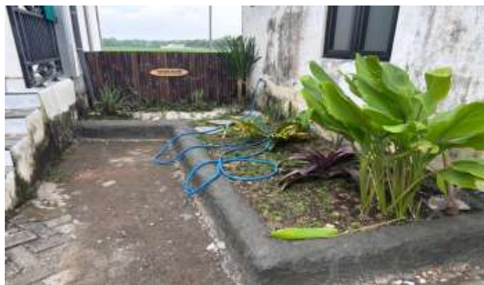
Figure 5. Final Condition of the Rain Garden as Active Green Infrastructure
