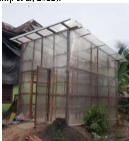
Figure 5. Polycarbonate kemplang drying house
